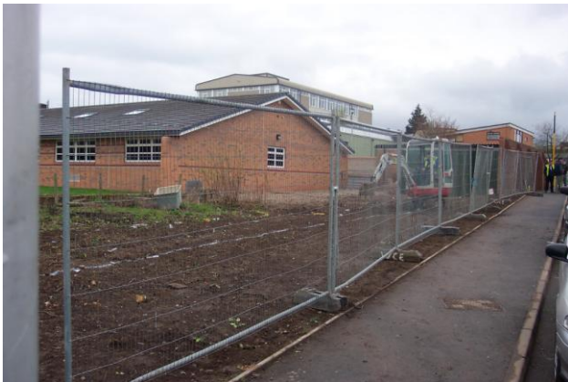
The school prior to the Green Barrier™ being installed.
