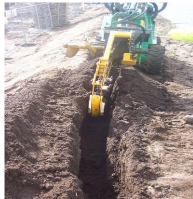
Excavating 600mm deep trench through the top of the earth bund.
