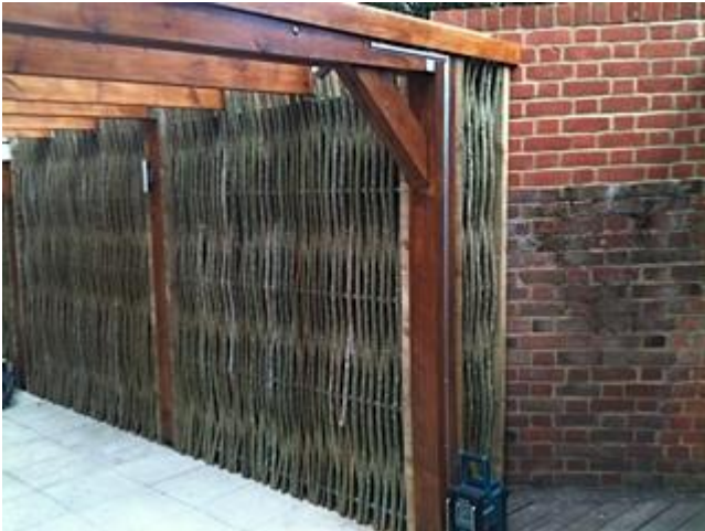
Insulation and woven willow panel against brick wall stopping noise reflection troubling neighbours.
