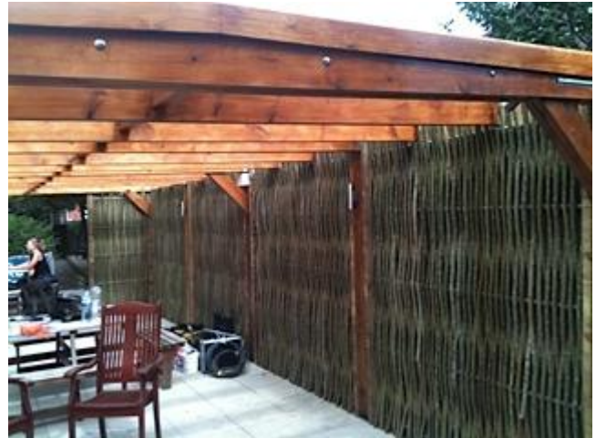
Insulation and woven willow panel against brick wall stopping noise reflection troubling neighbours.
