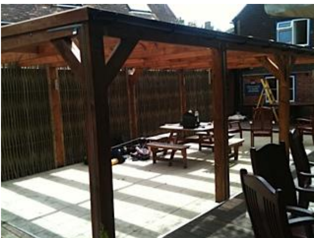
Insulation and woven willow panel against brick wall stopping noise reflection troubling neighbours.
