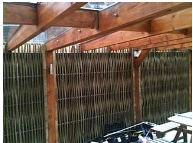
Insulation and woven willow panel against brick wall stopping noise reflection troubling neighbours.
