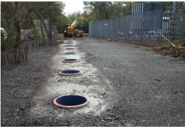
The ground prepared for the installation of the Barrier
